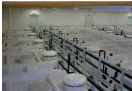
PVS VOPROM WWTP
