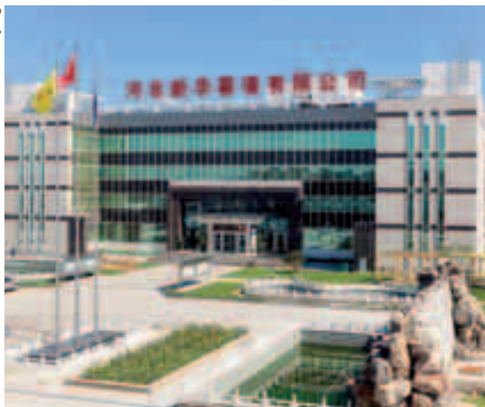
First office building in Passive House Standard China, Beijing
